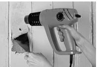
There is no way to eliminate dust, but some renovation methods make less dust than others. Contractors may choose to use various methods to minimize dust generation, including using water to mist areas before sanding or scraping; scoring paint before separating components; and prying and pulling apart components instead of breaking them.
